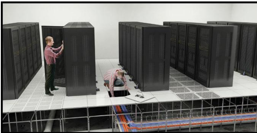
Figure 9 Raised Floor
